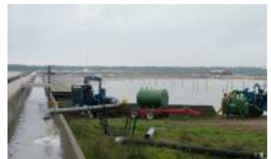
*Pumping Cell #4 down for sludge removal using our 12-inch pump*
