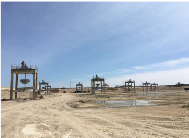
Cell two prior to filling.
