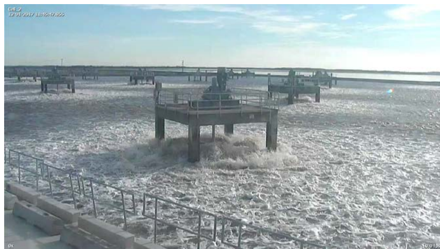
Cell two's new mixers
