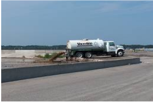
Figure 1 - Septic Hauler discharging into Cell #4
