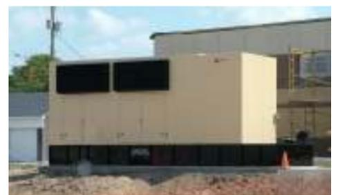
*1500 KW generator for new C Station*
