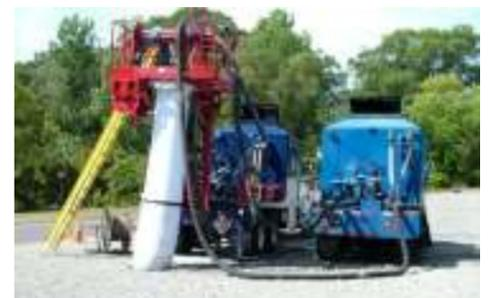
*Lining contractor installing pipe in Ruddiman Area Sewer*
