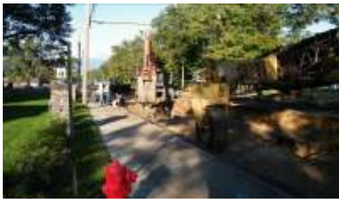
98% done! 60-inch force main installation approaching Harvey on Marquette
