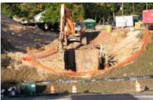
Boring pit for installation of the 60-inch pipe under US-31
