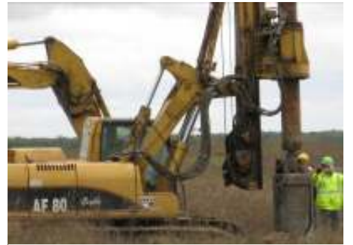
Drilling new gas wells in Landfill Cell #1
