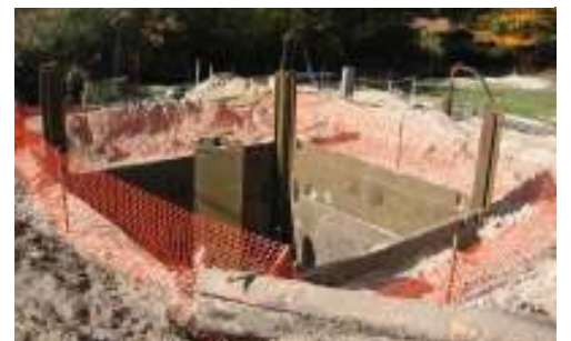
Excavation for Laketon Township sewer lift station
