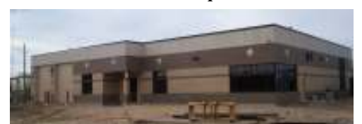
New Lift Station C almost complete
