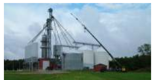
Painting of the 50,000-bushel bins and loadouts completed
