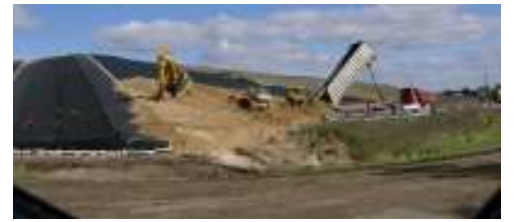
Covering the new liner at Solid Waste
