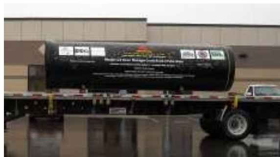
Signature pipe being moved from Lift Station C to Marquette Avenue for installation
