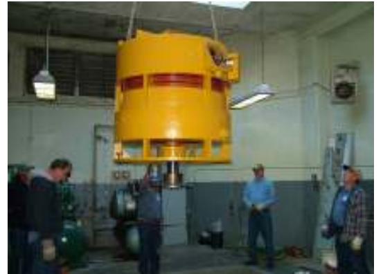
1,250 horsepower pump motor being placed back in old C Station
