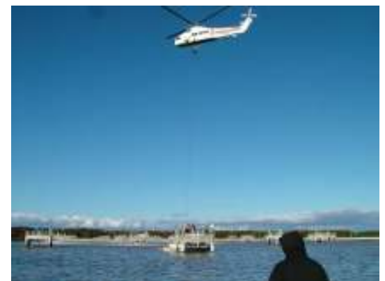
Pulling 100 horsepower mixer motors in Cell #2
