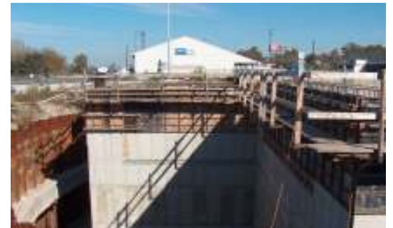
Forms up above grade now at our new Lift Station C
