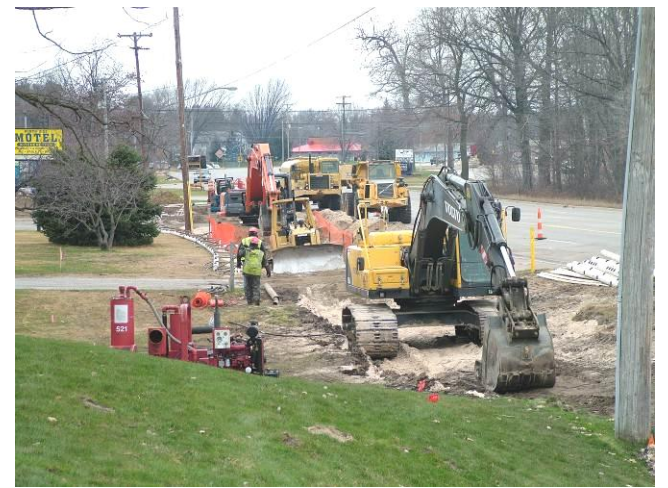
Work for the Laketon Township meter at Whitehall and Dykstra Roads
