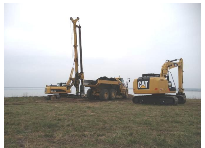
Landfill gas collection expansion work
