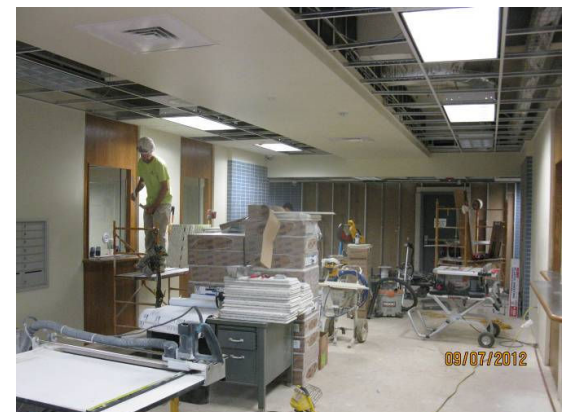
Renovation work on the first floor of the Hall of Justice
