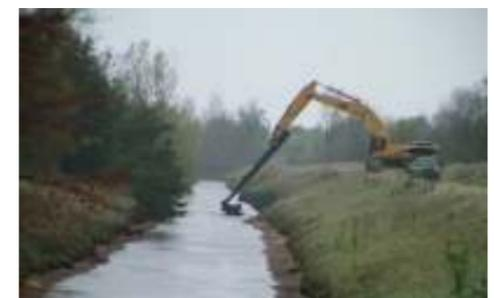
*Cleaning the sediments from the Laketon Station Ditch with our backhoe*
