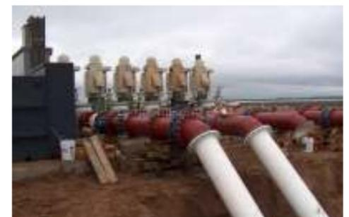
*Pipe work at Pump Station #3 as part of the strainer addition*
