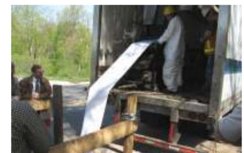
*John Warner observes liner being placed in water pipe on Quarterline Road*
