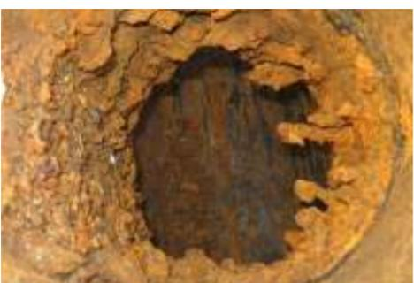
*Corrosion inside Quarterline Road water main tee*
