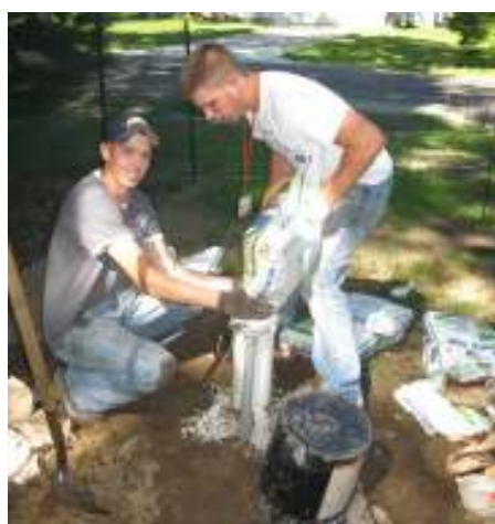
Well abandonment in Laketon Township
