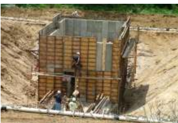
Walls poured at Sullivan Station
