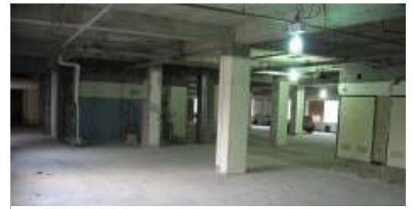
HOJ second floor is razed and ready for remodeling
