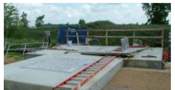
New concrete pad at Laketon Station
