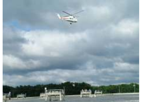
Helicopter moving gearboxes and motors from Cell #2 to Cell #1
