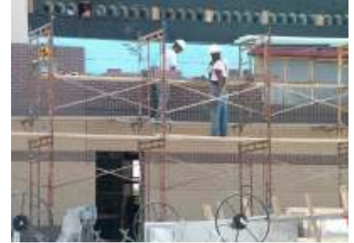
Brick being laid at C Station
