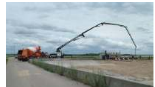
Pumping concrete at Pump Station 3 strainer project
