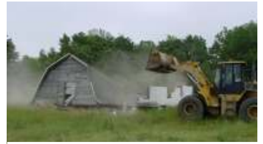
Barn demolition on Apple Avenue property
