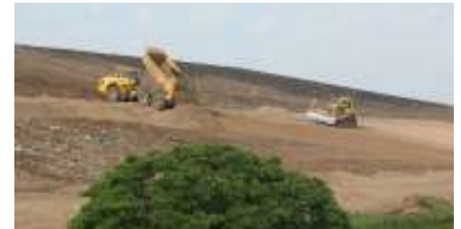
Placing the two-foot sand cushion on the landfill cap
