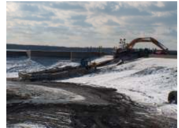
Sludge pumping from Cell #4 was finally shut down for the winter
