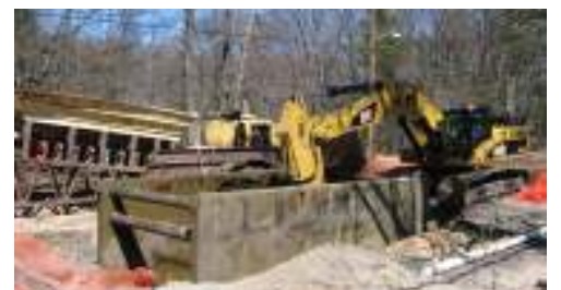
Laketon Township sewer installation on Pennsylvania Avenue
