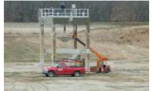
Placing new frames and rebuilt motors and mixers in Cell #1
